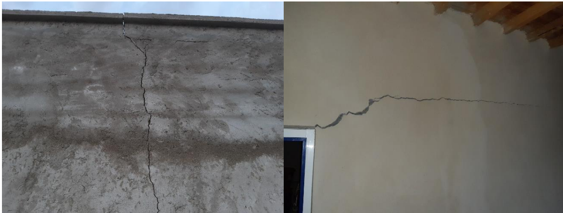
FIGURE 61. CRACKS IN THE WALLS OF THE HOUSES OF SORKHKUH VILLAGE
